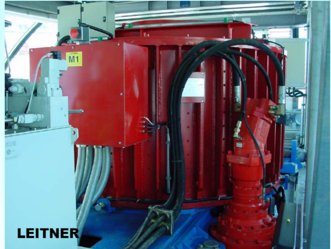
Synchronous PM excited motor as a direct drive with a tooth coil winding and a vertical shaft
