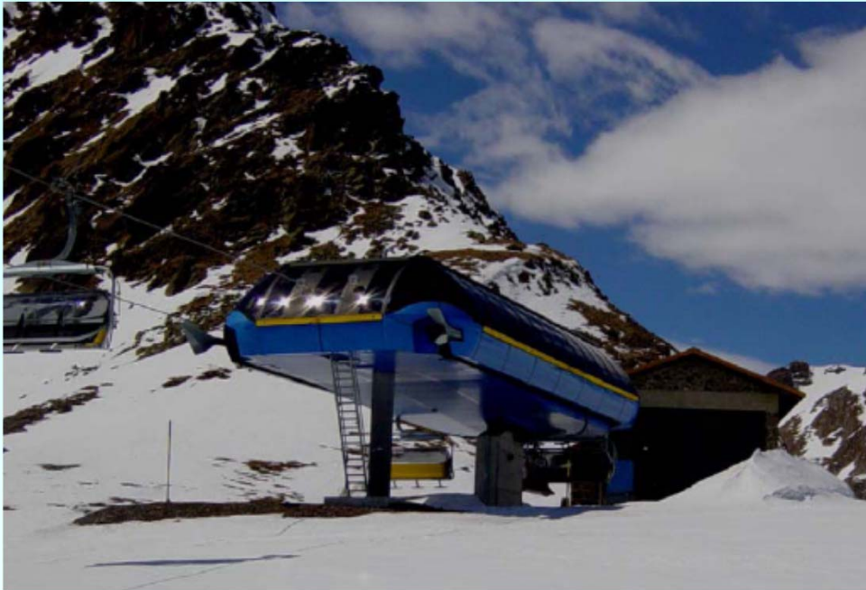
Mountain station of the cable car (for ski sports)
