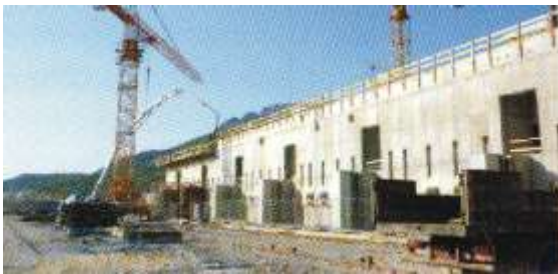
Ashta I building site
