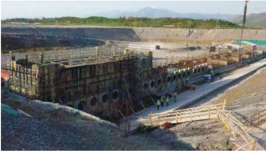
Ashta II building site
